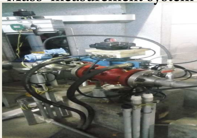
Fast diverting system
